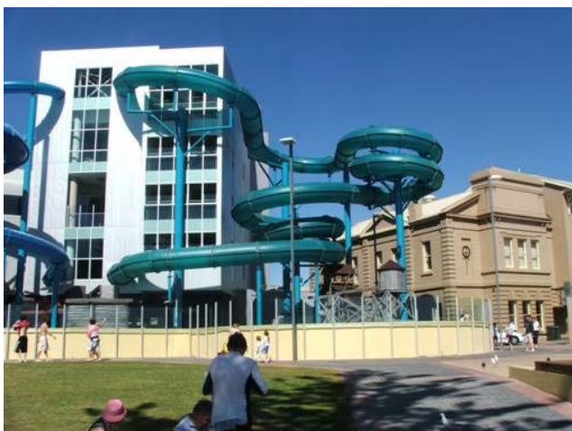
Beachhouse water slides at Glenelg
